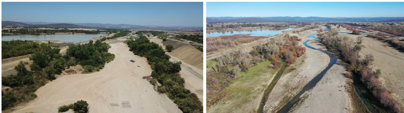
Figure 14: Left: Previously dry floodplain with “The Middle Training Wall” –a tall linear structure constructed by dredge miners to redirect the river’s flow. Right: The perennial channel now running through the floodplain that will, hopefully, be frequently inundated (Source: CBEC, Inc. Eco Engineering ).
